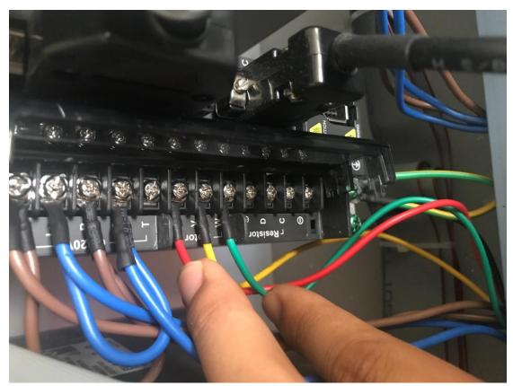
3. If the driver is marked Z1, find the same cable in B board with the
